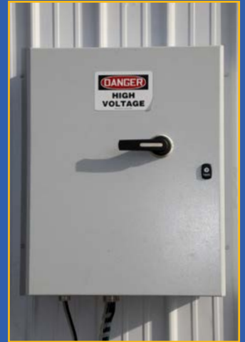
Exterior view of electrical enclosure box with 50' of wire between box and motor being standard which is sufficient for 30' tracks.
